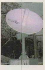
can receive signals from the satellites during the earlier (or later) stages of any particular pass. Signals in the 137MHz (v.h.f.) band are attenuated by physical obstructions, so generally, the height of the antenna dictates reception limits. Using good quality, low-loss, matched cable (usually 50 or  $75\Omega$ ) to feed your receiver, you should not require a pre-amp in order to hear the WXSAT signals.
