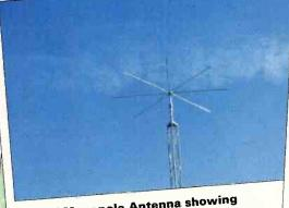
Top of Monopole Antenna showing capacity hat and loading coil.
