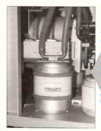
Vacuum capacitors used in the transmitters are watercooled. There's no shaft to turn the rotor plates here!
