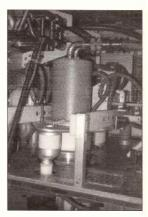
At the heart of each 500kW transmitter is a Thompson TH-55A valve. The watercooled valve has 30kV on the anode so the cooling water must have high resistance.
