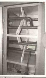
Shown here is one section of the ande inductor for the transmitter. Large diameter copper pipe ís necessary because of the high power levels involved.
