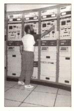
**Although the** transmitters can be completely controlled by computer, the technicians must be prepared to manually select the on/off time, frequency, appropriate antenna, antenna takeoff angle, antenna slew angle and programme. Each of the ten 500kW transmitters has a control rack. Four of the racks are shown here.
