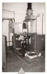
Dummy loads must dissipate considerable power. Shown here is one of the dummy loads. The black coaxial cable can be seen entering the dummy load at the top of the photo. The tapered metallic section below the coaxial feeder is an impedance matching section.
