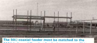
300 $\Omega$  balanced line that feeds the antennas. This may look like the initial construction stages of a bridge, but its actually a balun.
