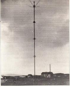
Machrihanish 122m tower and station showing the 'Umbrella Capacity' shrouds, insulated guywires, and ball and socket base.
