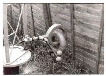
Toroidal transformer to feed mast lights. Plus discharge balls!
