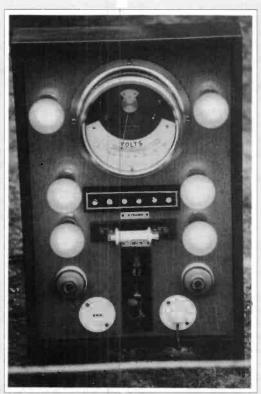
Fig. 2: A beautifully restored distribution board, originally used to supply low-voltage lighting in country houses.
