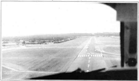
Approaching Runway 26L at Gatwick. The threshold is quite a bit beyond the apron. Note the glideslope antenna off to the left of the threshold, also the precision approach path indicator lights. *Photo Godfrey Manning*.
