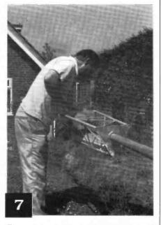
The rotator is housed in a galvanised steel cage which clamps onto the top of the upper section of the mast. Tennamast can supply cages drilled to suit any of the popular rotators. I used the rotator which had seen eight years service at the top of my pole. If you are using your old rotator then I recommend that you service it before bolting it in place - I didn't and the main bearings had disintegrated!
