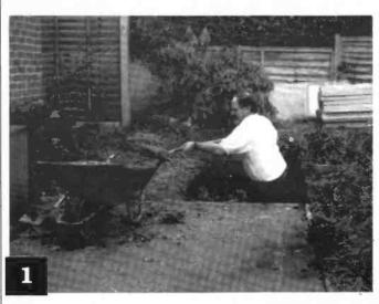
Apart from the mast and rotator cage, you will need a fine weekend,  $0.5m^3$  of  $3/_4$  in ballast, two bags of cement and some muscle-power. The ground post requires a concrete base 1 x 1 x 0.5m, so get digging! Keep an eye open for any drains, underground cables or pipes and position the centre of the hole far enough away from your boundary to keep the antenna from overhanging your neighbour's property and well clear of overhead lines.
