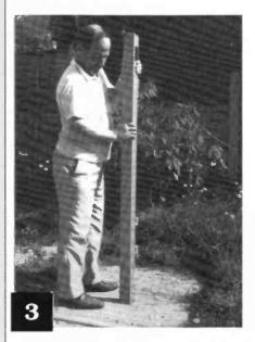
The ground post plugs into the socket - provided that you have kept it clear of concrete. Don't be too impatient the concrete needs several days to harden. Beware of frost in winter and protect the new concrete with a thick layer of sacking. In summer cover it with a polythene sheet to prevent it drying out too quickly. Before inserting the ground post into the socket smear thick grease all over the part of the post that will be in the socket.
