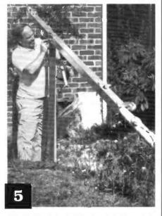
This is the bit that really needs an assistant (he had nippped off to take the picture). The main mast is lifted onto the ground post and the pivot boltinserted. The instructions suggest that a temporary support is used to hold the top of the mast level while you are doing this. In my case the ground sloped upwards so I didn't bother. The assistant will probably need to move the mast around to allow the bolt to slip in easily.
