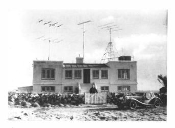
General view of the VHF beam installation at G5BY, Bolt Jail, South Devon, in December 1947. On the left, two wide-spaced 4-ele 58 MHz beams; a close-spaced 51 MHz 4-ele is at the centre with, on the right, an all-metal wide-spaced 50 MHz beam.
