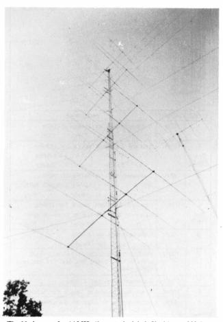
The 16-ele array for 14 MHz (four stacked 4-ele Yagis) on a 200-foot tower.
