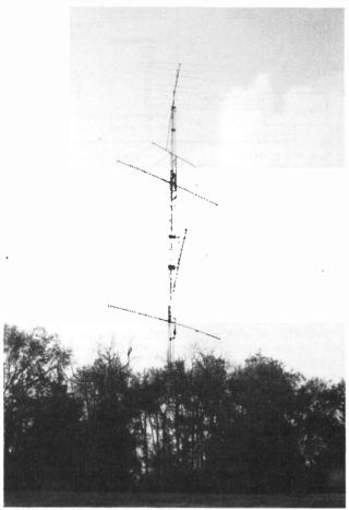
The 140-foot tower with stacked 5-ele Yagis for 14 MHz and stacked 4-ele Yagis for 28 MHz.
