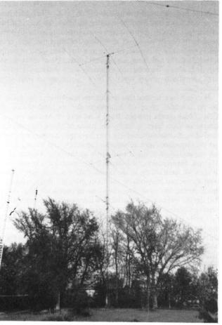
The 160-foot tower carrying the 3-ele Yagi for 7 MHz.
