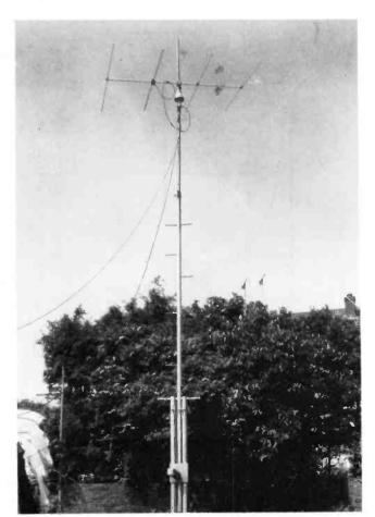
GW4BCD's homebuilt crank-up, tilt-over 45-ft. mast, with a 4-ele 6m. Yagi on top.
