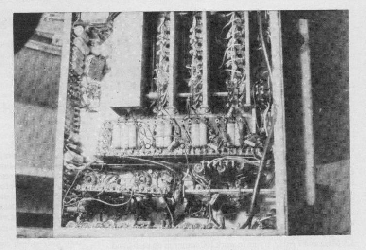
An underview of the receiver showing the coil pack and the extensive use of tag boards.
