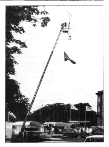
Sefton A.R.C. organised a special event station, GB4WMS, at Wigan Motor Show in June. Above, the 52-ft. multi-purpose 'mast', which sported a 19-ele Jaybeam for 70cm., 16-ele Tonna for 2m., and four 15-over-15 slot Yagis for 23cm. Below, some of the members of Sefton A.R.C. who helped run the station: back row, left to right, G8ZWZ, G8YPL, G61CR (Hon. Sec.), G6PZW, G4KIN, G6NRK and G6WFE. G6NIN (left) and G6EXC are at the front.
