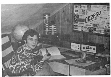
The mostly home-built 160m. station of Rostislav Pospisil, OK2PGU. Tx ] antenna is a 125-ft. vertical with a capacity hat, while a Beverage is used for receiving. Rosti, who already has 160/WAC, is aiming for DXCC/160—with 48C/43 so far in the bag. (Photo courtesy of W1BB).
