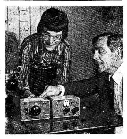
The West Kent Amateur Radio Society's Club Constructional Contest was won by G3XPX—with a small transmitter and receiver, conceived because somebody bet someone that it was not possible to work Europeans with just a torch battery for power. The Tx works on 80m. and uses four BFY52 transistors and incorporates SWR indication.
