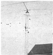
A self-supporting galvanised steel tower for HF band beams. Each 10' side weighs only 22 lbs., so the tower can be erected single-handed. Price: £47-00 carriage paid.
