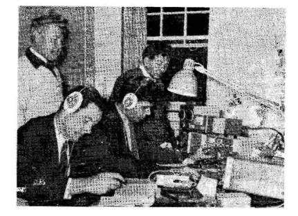
R.A.F. Abingdon Club Station G3TAB, operated by, left to right standing: G3KTC, G3MNN and seated G3XHK, G3VOD. They claimed 4281 points, using a KW-2000 /2E26A PA into a full-size 160m. inverted-Vee with the apex at 90ft. This picture well conveys the tension and excitement MCC engenders when the operators are taking it seriously.
