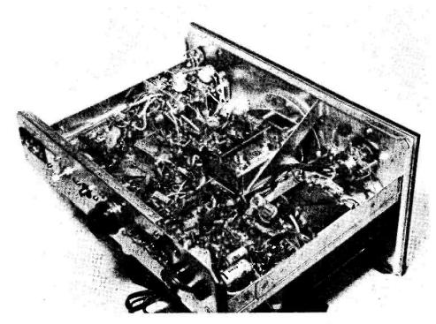
General under-chassis layout and construction of the Trio JR-500. Again the 160-metre modification is not easy to pinpoint but is involved in the wiring beside the coil pack at upper left. This modification can be applied only by the suppliers (in this case Holdings of Blackburn) for customers taking new receivers.
