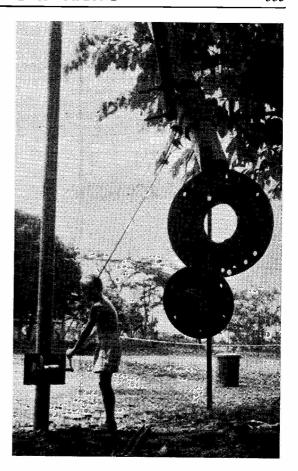
The heavy pieces of iron are hung on temporarily to counterweight the mast, reducing the top-heavy weight to about 30-40 lbs.—making it possible for young 9L1HX (junior) to haul up Dad's 20-metre Quad on its 60-foot mast—see text.
