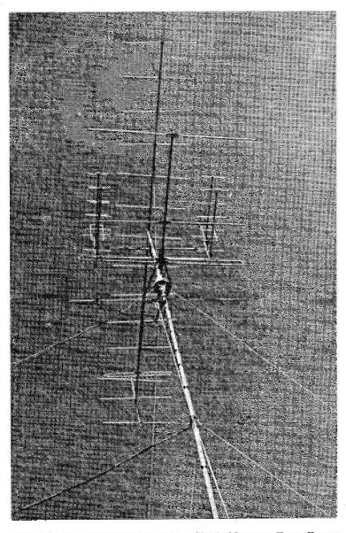
VHF aerial set-up at EI6AS, Dublin, who is ex-G3JLA of Stevenage, Herts. Here we see a 13-ele beam for two metres, at 44ft. (upper array). Below that is a 6/6 Yagi for 70 centimetres, the 430 mc band. Underneath is a 4-element beam for four metres. The whole lot is turned by a CDR rotator. Now fully equipped, EI6AS is competing for Eire on the VHF bands.
