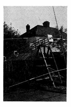
(B) A seven-feet high support cradle, or "launching pad," was made for the G3SM 40-feet tower, here seen ready to go up with the TA-33Jr. beam in position.
