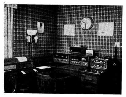
W6AEE, 372 West Warren Way, Arcadia, Calif., has an HT-32A/33A transmitter and SX-117 receiver, with his own design of terminal unit. The printer is described as "ASR-28, home assembled from parts." The signal is radiated off an all-band vertical aerial system.
