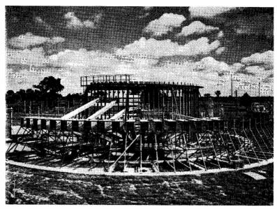
What an aerial switching panel for a QRO broadcaster can look like — the outdoor unit, under construction, for switching ten of Radio Australia's high-power HF-band transmitters in conjunction with a 36-aerial system giving directional coverage to all parts of the world.
