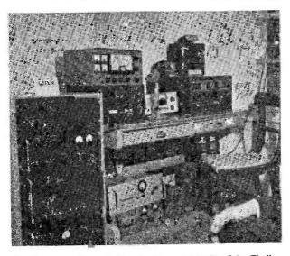
The two-metre station of G3JXN, operated by Dr. John Tindle at .149 Hamilton Terrace, St. John's Wood, London, N.W.8. The QTH is actually a block of flats, and G3JXN has his slot-fed 6/6 on the roof. Right is the two-metre PA, a QQV06-40A running 100w. and modulated by a pair TT21's. G3JXN was one of those who knocked off HB1ADT during the late-July opening, and he is now at 12C in Countries Worked. Prints by G3AWS
