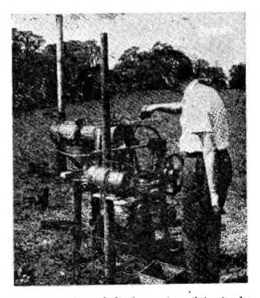
Rather unusual (to say the least) power generating system for the Loughborough Club's recent field day — a miniature steam plant driving a 230v. AC generator. For the consumption of only 1 cwt. of small coal, the little engine ran non-stop for 24 hours and gave a steady line voltage with sufficient amps, for the whole station. The plant was provided and supervised by Mr. George Wall, a local model engineer and friend of the Loughborough Club group.
