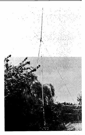
An impression of the G6AS three-band vertical radiating system; the guying is at 30 ft., and the mast is extended to 41 ft. with an 11 ft. whip. Three plastic cord guys at 15 ft. spread from the base of the radiator give ample support, and the mast also holds up one end of a horizontal aerial.
