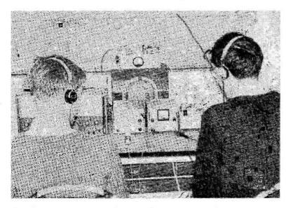
The VHF station at the Ministry of Aviation site on the summit of Snaefell, I.o.M., with G3RSE in front of the 4-metre gear (lent by the Pye group) and SWL Burden (left) doing the logging. GB3CUW was the callsign on four and two metres, the gear for the latter band being Withers throughout, with an Eddystone S.940 receiver as IF/AF strip. Some 17 stations were worked on 4m., and 45S on two metres.
