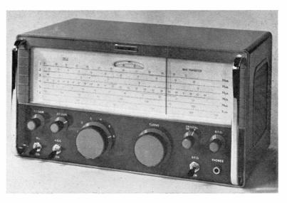
The Eddystone 960, seen on the stand of Webbs Radio at the Seymour Hall Exhibition this year, is a very interesting design in that it is all-transistor, tuning 500 kc to 30 mc in six ranges, and has a full communications specification. The power supply is a 12-volt battery.
