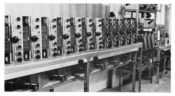
Part of the production line at the K.W. Electronics, Ltd. works at Dartford, Kent, showing a batch of the new KW-77 receivers. On view at this year's Amateur Radio Exhibition, these are now coming off regularly, for orders from all parts of the world. The KW-77 has excellent characteristics for specialised amateur-band operation, is of outstanding quality, and is rapidly making a name for itself. It also has the advantage of being reasonably priced for its class.
