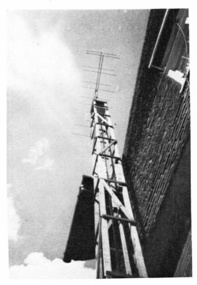
General view of the G6US lattice tower, in position with the 6/6 J-Beam at a height of about 40ft. The article describes its design, construction and erection in detail.
