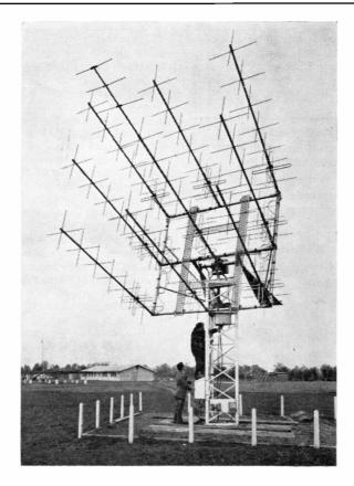
The remote-controlled steerable Yagi array at the Winkfield station of the Radio Research Board, and now in use for keeping in contact with the U.K. satellite "Ariel" on 136.41 mc. Eight of the 3 x 3 sections are phased to work as the receiving aerial for the satellite {-watt transmitter ; the ninth section, in the centre, is for transmission to "Ariel." The whole array is controlled from the Winkfield operations room.
