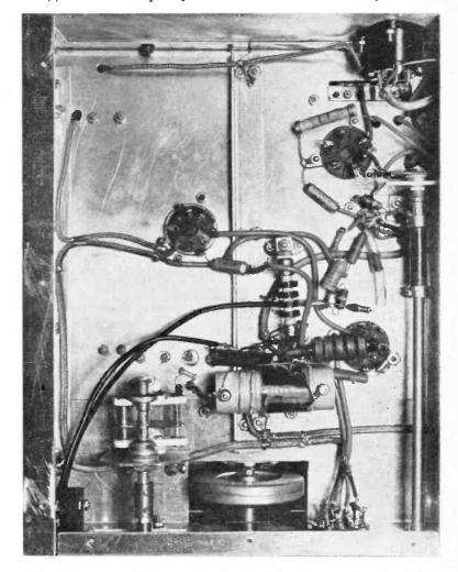
Under-chassis view of the Frequency Meter, showing general layout. The switch S2 (see circuit) is beside the dial-control flywheel, and the zero-setting condenser on the left of the coil. The power connections are carried in screened leads.
