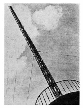
Dexion is well known as pre-fabricated constructional material in strip form. Here is a 60 ft. tower built throughout of Dexion.
