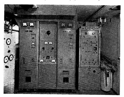
The central assembly consists of the two NT203 wideband RF amplifiers, which can be operated in parallel; between them is the control and monitoring unit. The transmitter on the right is the NT201, which can be used either by itself as a 1 kW spot frequency Tx or, from its low-level stages, as a driver for the NT203's, which in parallel give a p.e.p. of 2.8 kW. These transmitters are remote-controlled from the operating position, to which monitoring indications are repeated.
