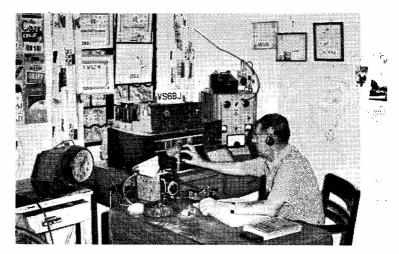
VS6BJ is one of the Hong-Kong group, located at Kowloon, and has an interesting station. The receiver is an AR88 and the transmitter a Labgear LG.300. For SSB working, he has a home-constructed half-lattice exciter with an 829B as PA.
