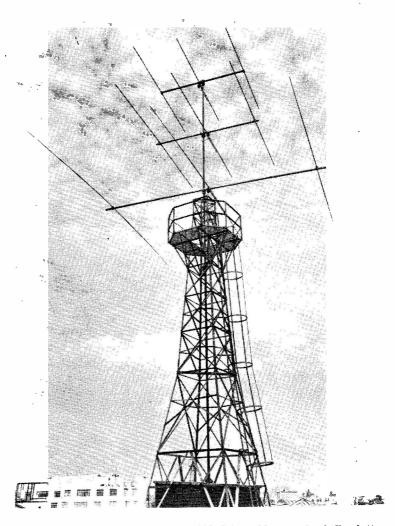
Three-band transmitting array for GB2SM, Science Museum, South Kensington, London, S.W.7. The tower, supplied by British Insulated Callender's Cables, Ltd., is 48 ft. over roof level, putting the 10-metre section of the array about 160 feet above the pavement. The other two sections are for 15 and 20 metres respectively. Having a separate, properly matched and fed, beam for each band has given GB2SM a muchimproved DX potential.
