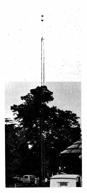
The aerial for G3GPW/P, the 160-metre control station for the Cheltenham Rally on May 10, was provided by G8ML of Francis & Lewis, Ltd. It consisted of a 70 ft, mast standing on a base insulator, with a top loading section known as a "parrot cage," making a very effective vertical transmitting aerial for Top Band.
