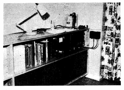
As this photograph shows, the TCS equipment makes quite a neat living-room installation. G3LOX has a BC-453 run as a "Q5'er" to improve the receiver side, as explained in his article, which gives a lot of practical information on the TCS assembly. The power supply and auxiliary audio amplifier (see Fig. 3) are in the lower cupboard. In effect, G3LOX has his whole station fitted in a book-shelf, the top of which serves as an operaing table.
