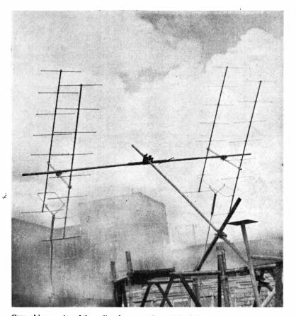
General impression of the radio telescope at Stowe School, Bucks., built up by G3HMO for operation on 200 mc. The array is set on an equatorial mounting, so that the sun can be followed round without any adjustment in elevation being necessary. The aerial system itself is described in the article. Very good results are being obtained, and large "noise signals" have been recorded when the sun is normally active. Noise has also been received from the Milky Way.
