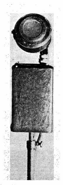
Microphone and head amplifier on its stand, complete, as described in the article. The increased audio gain enables the microphone to be "talked at" in comfort from several feet away, while allowing a connecting lead of any convenient length into the speech amplifier proper.
