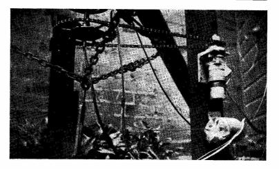
Base mounting and beam rotation gear at G3GSO, Derby. The head is a slot-fed 4-over-4 which, compared with the old 4-ele flat top, is giving very good results on two metres.
