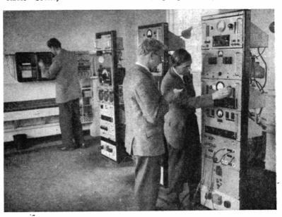
The receiving equipment for the Radio Telescope in operation near Cambridge. One of the items in the far rack is an R.1155. (From "Mirror in the Sky").
