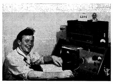
The station of G3JYS, Coventry, is a neat writing-desk layout, with a home-built CW transmitter operated on the LF bands.
