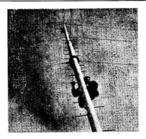
Mast and aerial inspection is a routine maintenance task in Antarctic territory, where 100 m.p.h. gales are usual. The masts are 70-feet high, supporting a variety of aerial systems. Here is VK1EG doing his stuff.
