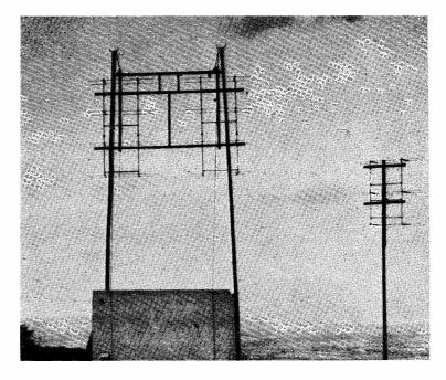
The 32-element fixed-direction beam at EI2W (Dublin), specially built and orientated to radiate on the heading for Scandinavia. Supported between two poles, it can be raised or lowered easily by means of a rope-and-pulley arrangement. To the right is the 12-element beam in normal use at EI2W for general coverage. This photograph gives a good impression of the clear get-away from the EI2W site.
