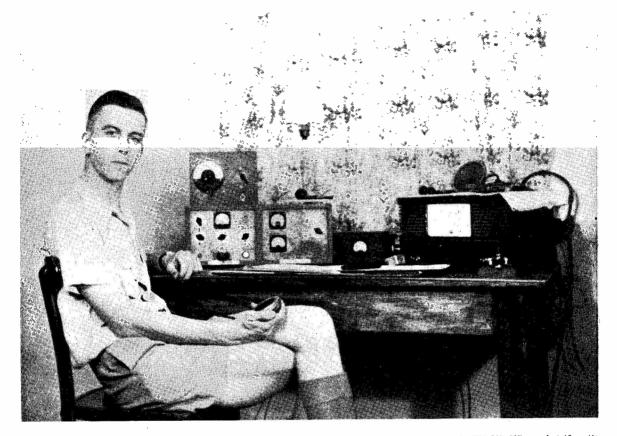
Station of ZE3JJ, Salisbury, Southern Rhodesia, who has been on the air since early 1950. The Tx is 6V6-807-807 running 60 watts, with optional CC or VFO control using a TT11 in an ECO circuit. Modulation is by a pair of 6L6's, and the aerial for Ten a 2-element rotary beam ; on the 21 mc band, ZE3JJ gained the world's first WAC, using a vertical Zepp. The Rx is an Eddystone S.640.
