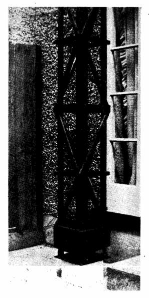
Photograph C. Showing the base assembly, consisting of a steel plate on a concrete block. By removing the two rear bolts and loosening the front pair, the tower can be lowered with the foot pivoted about these bolts.
