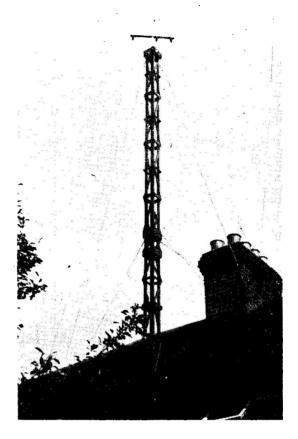
Photograph D. An impression of the whole assembly, as constructed and described by G3SM in his article, showing the guy-wire layout.
