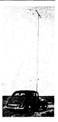
The neat /P set-up operated by G5MA on his portable expeditions. Everything is in or on the car, making possible a single-handed job. The beam is a 4-ele. Yagi, and the mast extends to 6 feet. This photograph was taken on the occasion of the GW5MA/P excursion to Llanybyther, Carmarthenshire, April 12-13 last.
