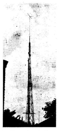
The G5YV beam head at the 62-foot level—still with 30 odd feet in hand to wind up. In other words, the beam can be pushed up half as far again? The "thickness" up the mast (which actually tapers gracefully and is a first-class engineering job) is a 42-ft, pole in the background which happens to coincide with the camera angle.
