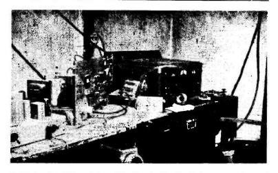
ZC1AZ as operated at Amman, Transjordan, for the two years to January, 1950. An 813 PA produced the RF on 14 and 28 mc, CW and Phone, with a pair of 805's in the modulator. Receiver was an SX-28, aerials various (including a beam for Ten), and the operator of ZC1AZ is now G3GTA (Bath).
