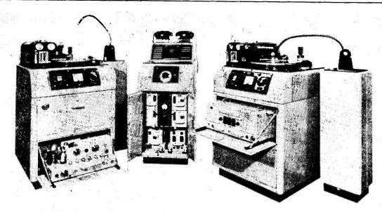
The BBC's Type D Recorder, as manufactured by E.M.I. Factories, Ltd. This is fine equipment for precision work of the highest order and is extensively used for BBC canned programmes.
