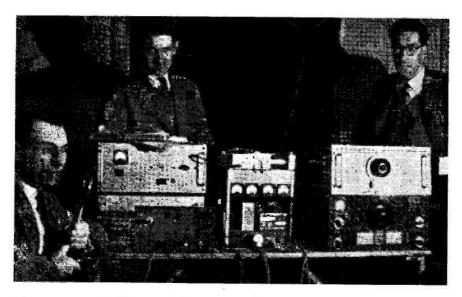
A 70 cm set-up at G3ASR on April 18 last, when a Seventycem demonstration was given to the Edgware Club "for one night only." G2DD is on the microphone and the 70 cm transmitter is in the centre of the array of gear.
