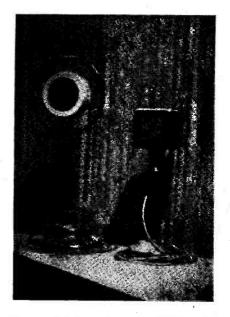
Two microphones produced by G5WW on the principles discussed in his article. That on the left is in a circular container which at one time held a high wattage resistor. The microphone on the right is built into a rectangular metal box and the stand is adapted from an ex-A.M. "candlestick" telephone.
