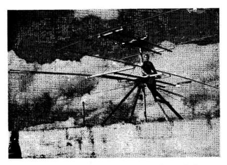
The rotary beam assembly at ZBIAH, Malta, for operation on Ten and Twenty. The 28 mc section is 3-element and that for 14 mc is two elements.
