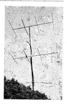
Dual 4-element wide-spaced beam stacked and fed in phase, G4CI, New Malden. Surrey. Radiators are arranged to present 100 ohms at their feed points, individually. The ½-wave section toining them has a surge impedance of 155 ohms; this operates as two independent ½-wave sections giving an impedance rise up to 200 ohms at the point where the feeder is connected.
