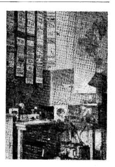
The outfit at ZBIAR, Malta, a 25-watt station. Tx, at left, is VFO-Tritet, into a pair of 807's in push-pull or push-push for the 7, 14 and 28 mc bands.
