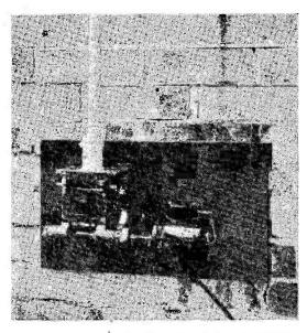
Gearbox and motor assembly for rotating the beam at G2HNO. The box has slip rings for use with a coaxial feeder taken up inside the supporting mast.
