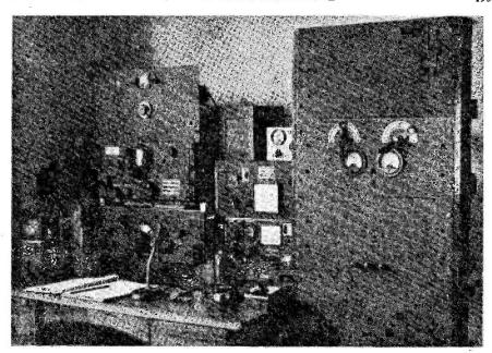
G3AST, Luton, Beds., is operated on 7 and 14 mc. The Rx with an HRO dial is a 16-valve home-built communications superhet with plug-in coils, and a BC-348 is also available. The Tx is 807-35T, with an RC-coupled speech amplifier-modulator running a pair of 845's in Class A.
