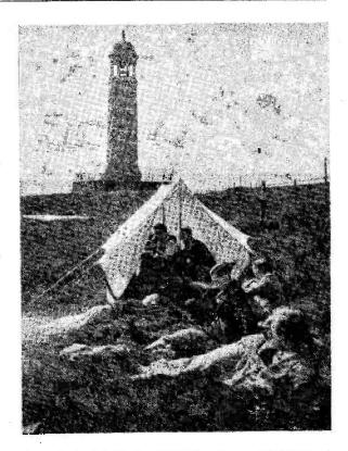
The lighthouse supports the far end of a 1.7 mc ½-wave aerial (264 ft.), and the operators on this station worked in shifts.
