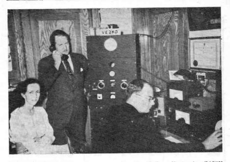
General view of VE2KG, Quebec, with ex-G2CIN at the operating position. The Tx runs 50 watts, using a 6L6-RK39 combination, into a 4-element beam.
